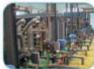
连云港田湾核电站 Lianyungang Nuclear Power Plant
